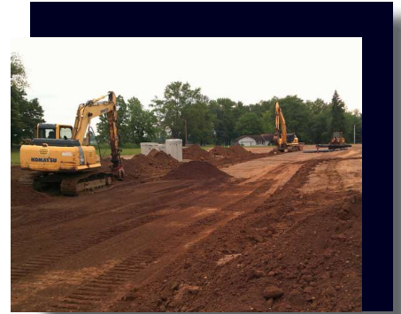
Wicker Creek No. 6 Road Base & Waterlines, Plain Township
