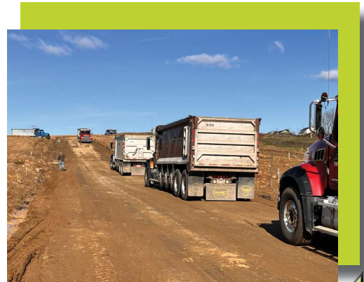
The Farms at Enclave No. 2 Truck Hauling Roadway Stone, Lake Township
