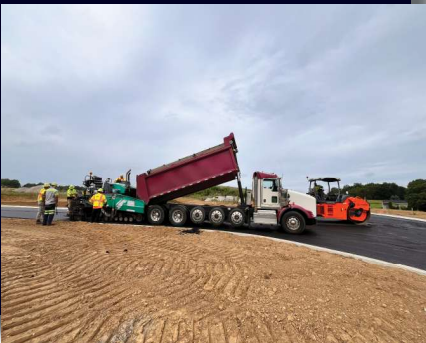
Weston Place No. 1 Paving Road, Perry Township
