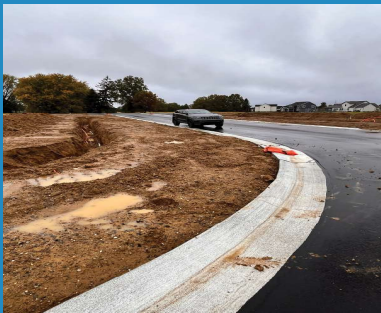
Rolling Green West No. 4 Private Utility Trench, Jackson Township
