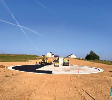
Oldestone Crossing No. 4 Paving a Cul-de-Sac, Lake Township
